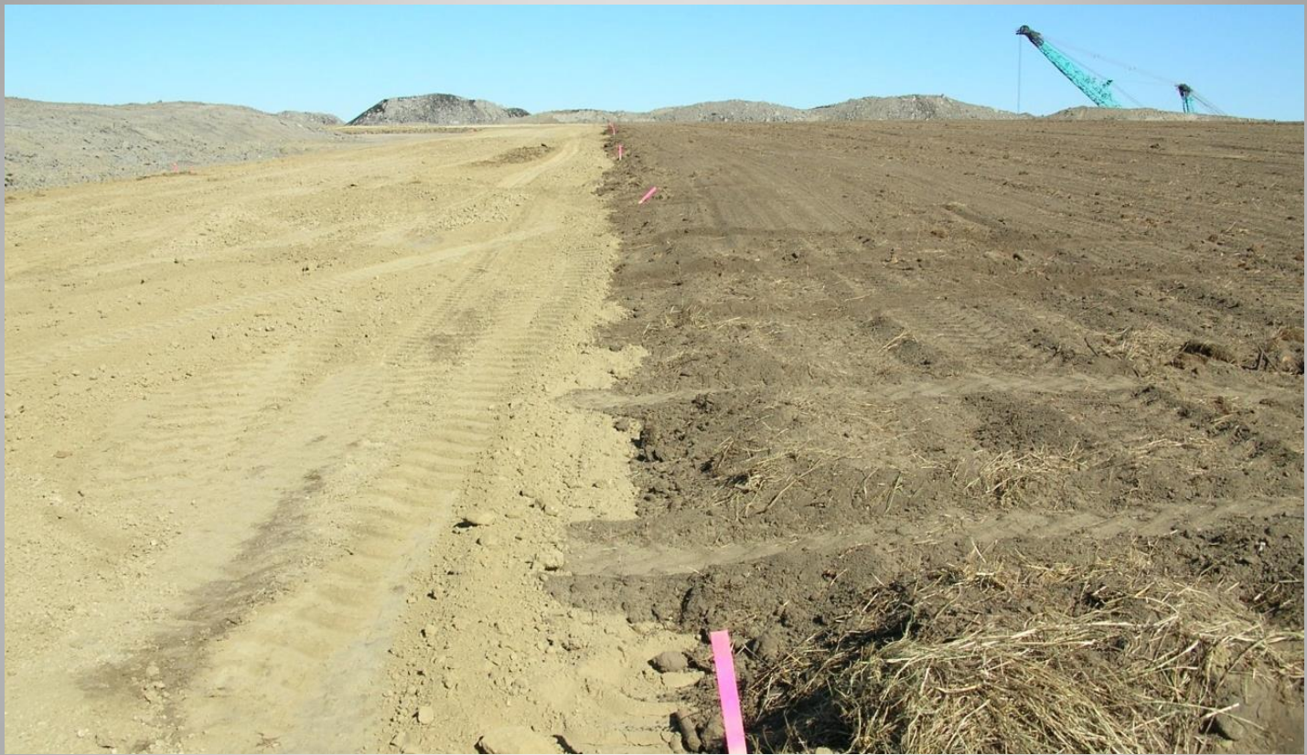
Recently respread topsoil and subsoil at the Center Mine
