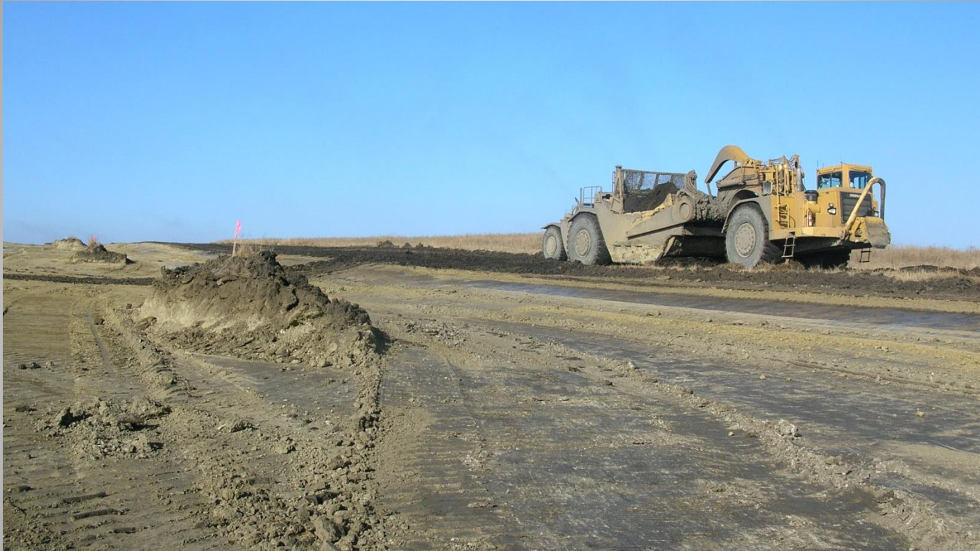
Topsoil removal with a twin-engine tractor scraper at the Center Mine
