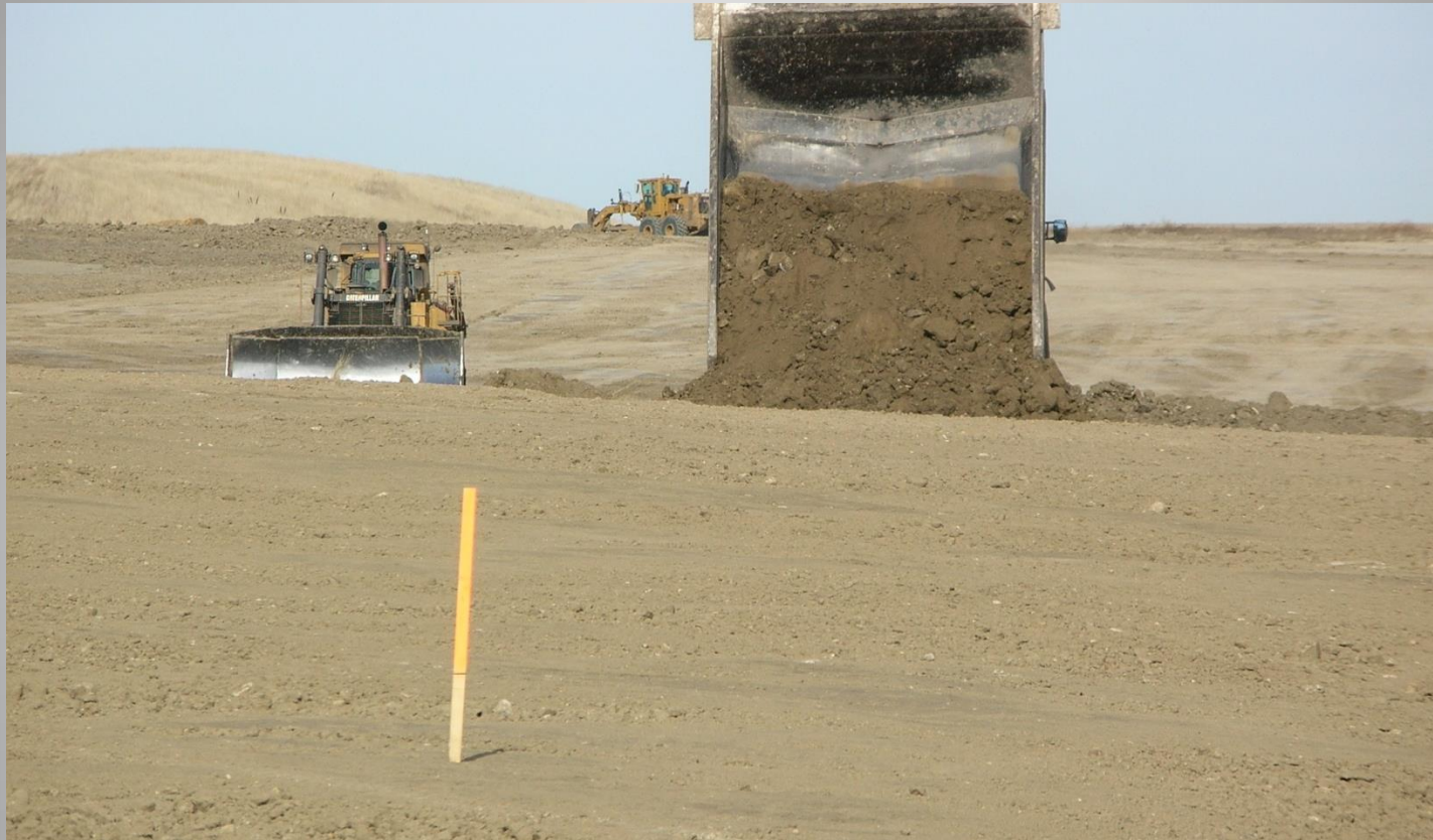
Subsoil being respread on graded mine spoils at the Freedom Mine
